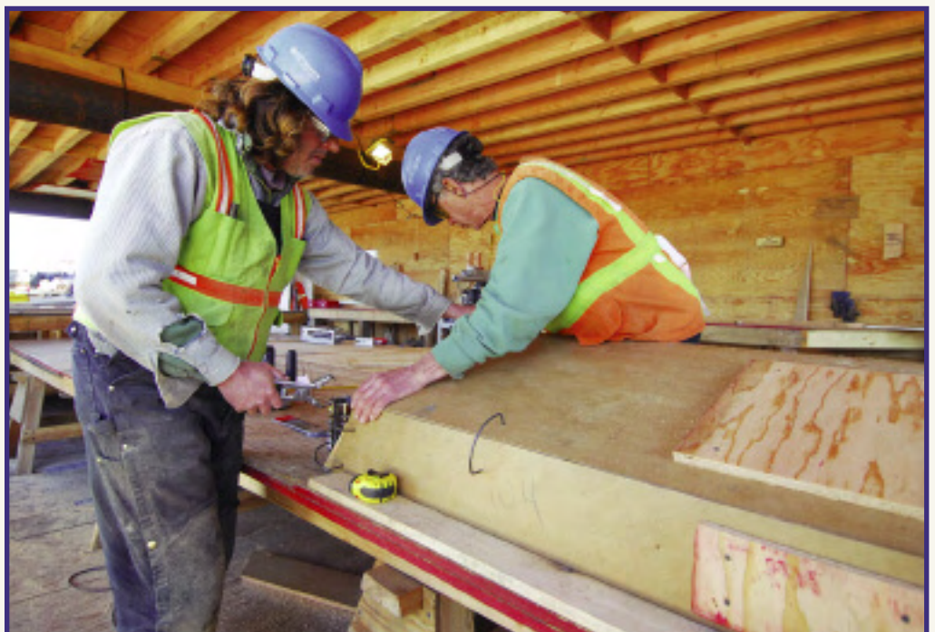
Tony Creighton and George McNeil building blockouts in K-M’s specially designed woodshop.
