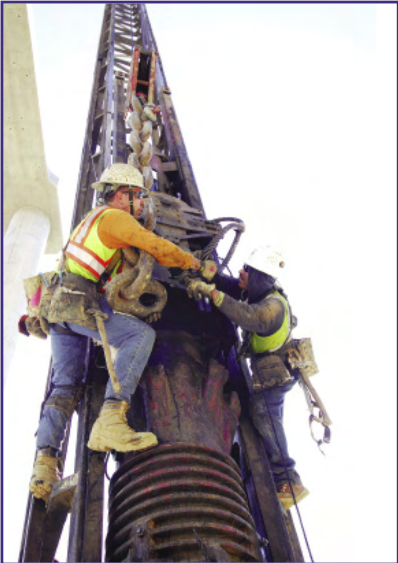
Scott Hale and Martin Espinoza rigging pile-driving hammer.
